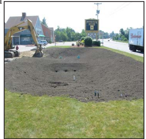
Bioretention Area During Construction
