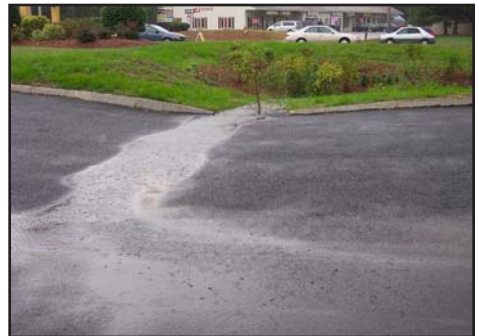
Precipitation Entering Bioretention Area from Parking Lot
