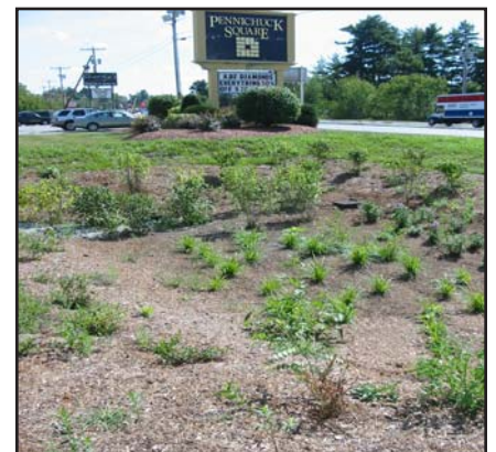
Bioretention Area After Plantings
