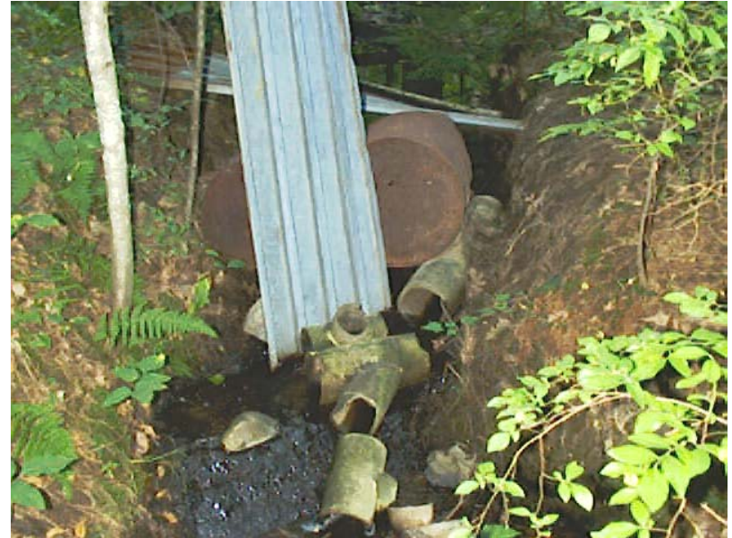
Figure 3-8. “Drum Bridge” Located in Stream Next to the Old Construction Materials Storage Area. This Stream is a Tributary to Bowers Pond.
