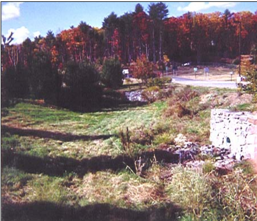
Figure 2-13. Postal Service Detention
