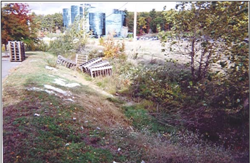
Figure 2-9. Northern Perimeter Swale
