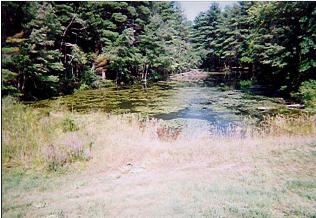
Figure 2-14. Controlled Outlet to Harris Pond
