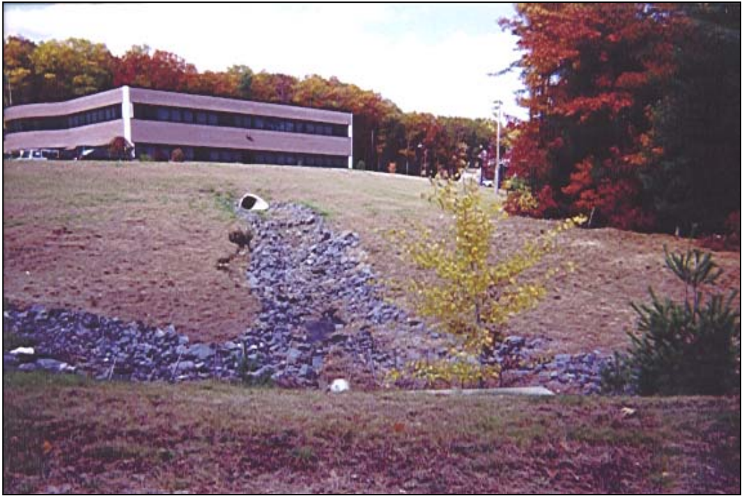
Figure 2-18. Stormwater Collection Junction for the Cornerstone Site
