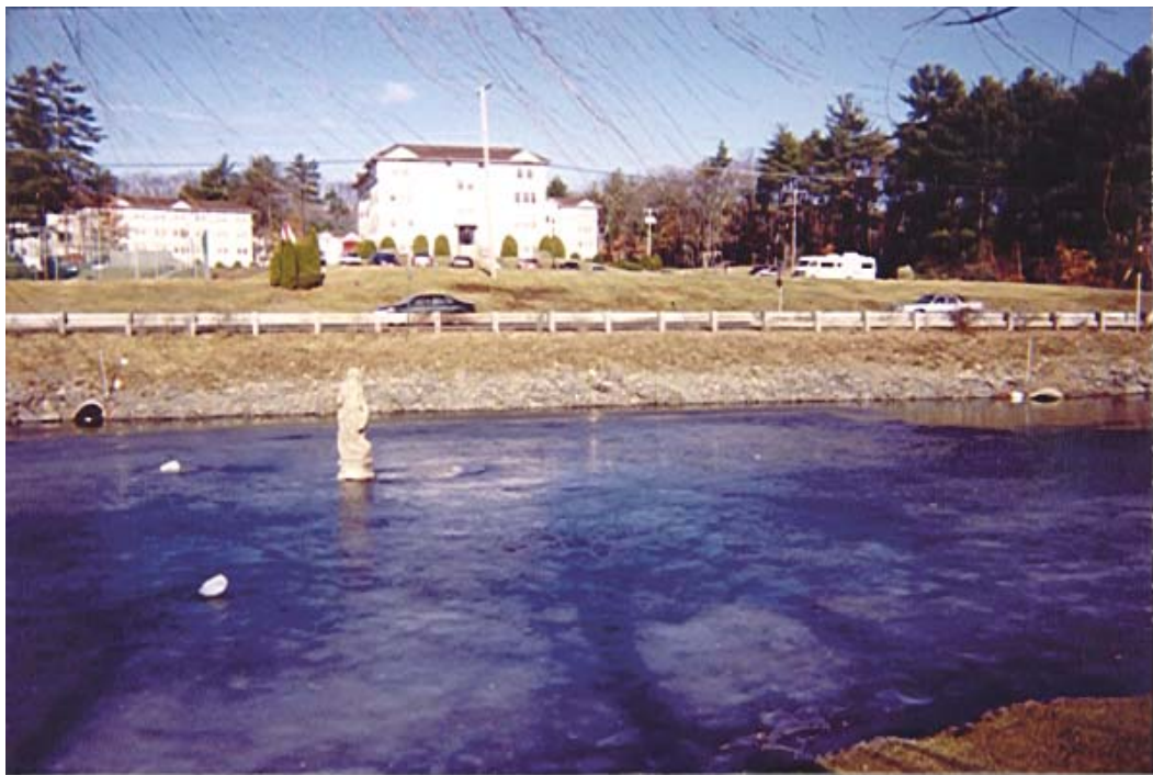
Figure 2-5. Stormwater Discharges to Crowne Plaza Detention Pond
